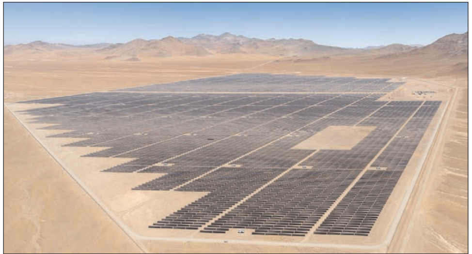
The Luz del Norte photovoltaic power plant.
