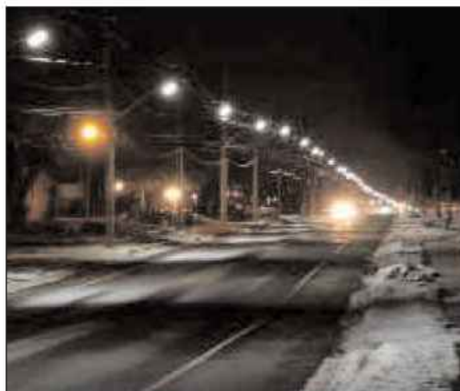
The 50 LED streetlights installed on Fitch Street, Welland, Ontario.
