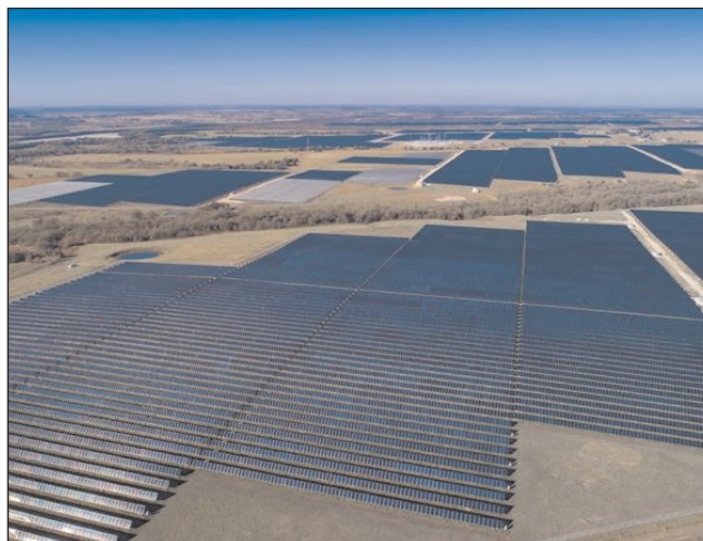
The 163MW Elm Branch solar power project in Texas was developed by Lightsource bp and is powered by First Solar Series 6 photovoltaic modules. (Photo: Lightsource bp)
