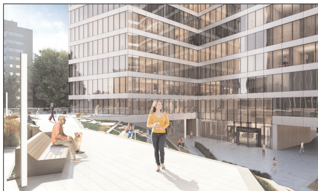
Example of Skanska's office building covered by semi-transparent perovskite solar modules. Perovskites are integrated into the property's façade without changing its design and aesthetics.
