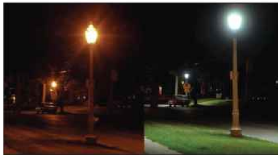
Conventional (left) and LED (right) streetlamp in Lansing.
