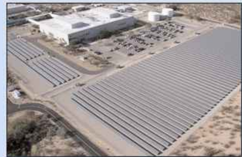
p57 Global Solar Energy has begun operation of the 750kW CIGS PV array at its 40MW plant in Tucson, AZ, USA.
