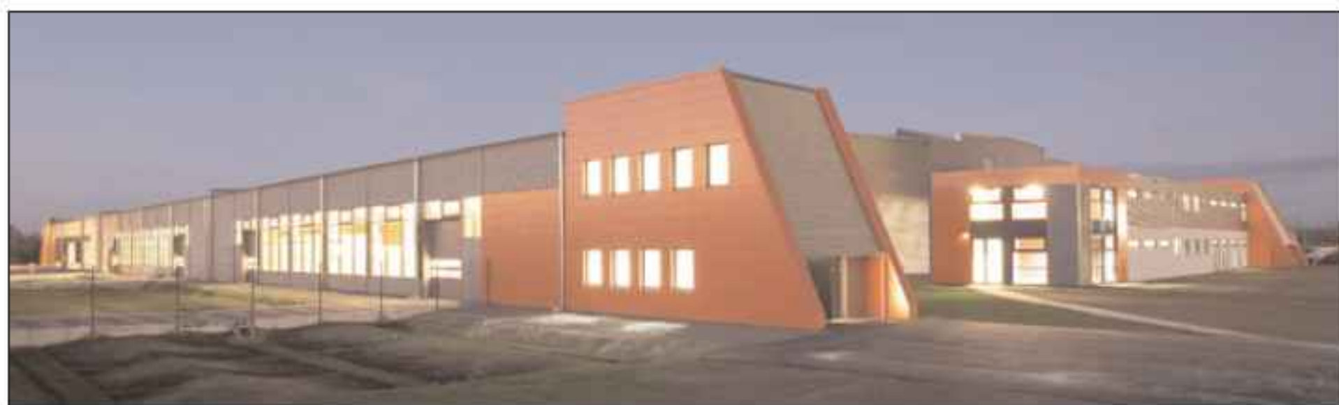
Johanna Solar's CIGSSe thin-film PV module manufacturing plant.
