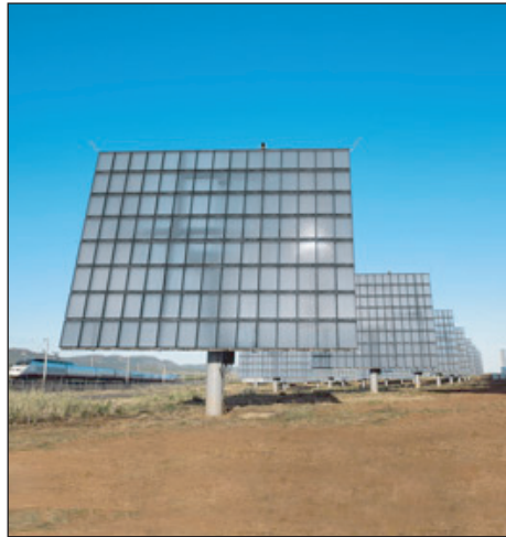
Soitec's Concentrix CPV systems.
